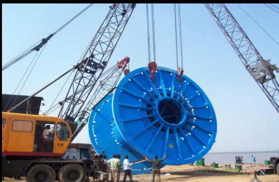
Lifting of Cable reels onto barge
